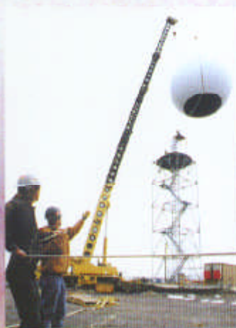
Radome construction and installation
