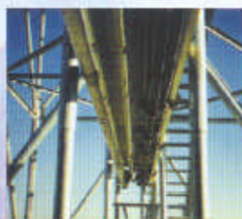
Coaxial cable and antenna installation
